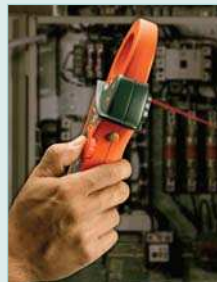
Built-in IR Thermometer with laser pointer is an excellent roublshooter for locating hot spots and overheating motors.
