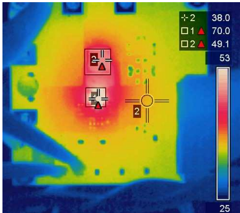
Fig. 17: Thermal Image (IR3473: 70°C, Inductor: 49°C, PCB: 38°C)
